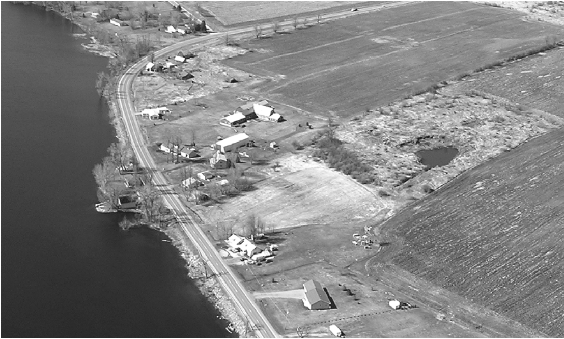
The quarry at King's Bay. This small quarry supplied stone used during the earliest stages of construction. Photo courtesy of Doug and Roger Harwood.
